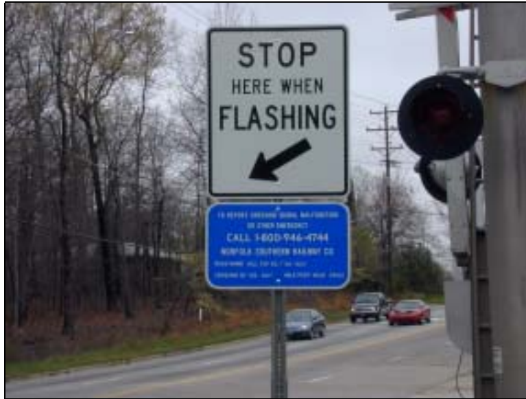
Figure 4.4 – “Stop Here When Flashing” Sign & Emergency Notification Sign (Hilltop Road)
